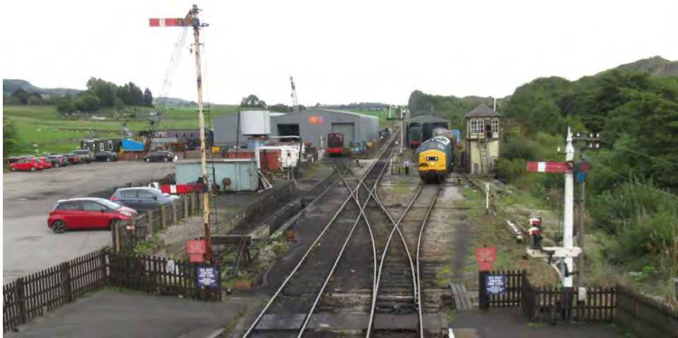
Emsay station signal box and yard
