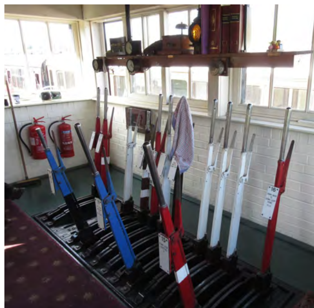
Inside Stoneacre signal box
