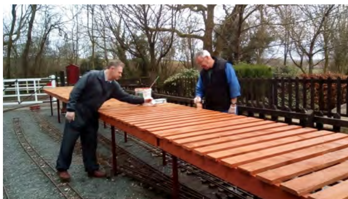
Once the frames had been boarded out the timber work was given a second coat of wood stain
