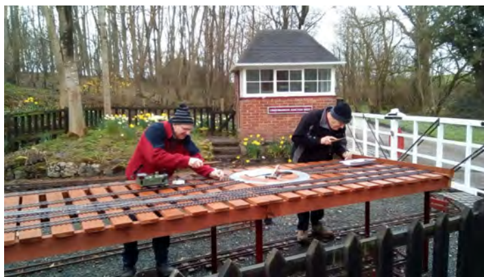
Geoff and Stan nailing down the final track. The area between them is where the turntable sits.
