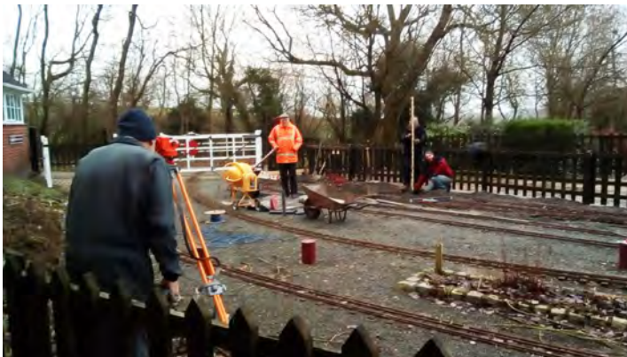
Leveling and setting the sockets into the ground for the steel supports
