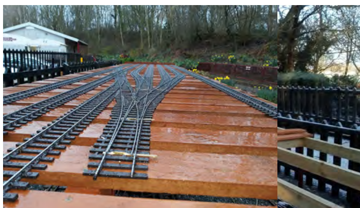
Track part laid and looking down the three-way point to the Marshalling yard, rain stopped play
