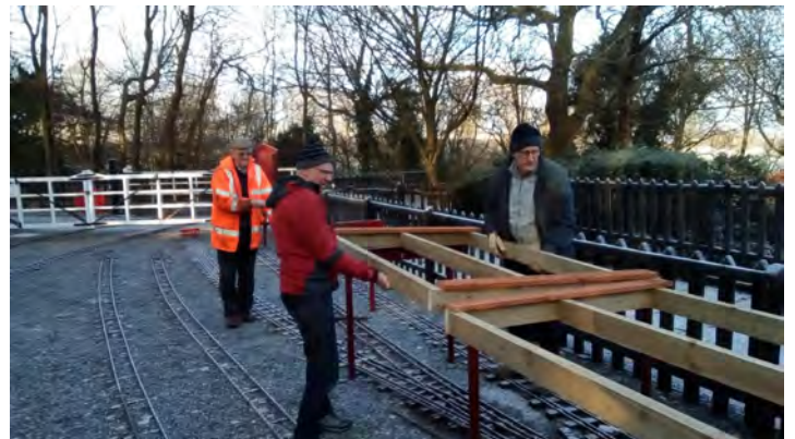
One crisp frosty morning the frames being test fitted between the metal supports
